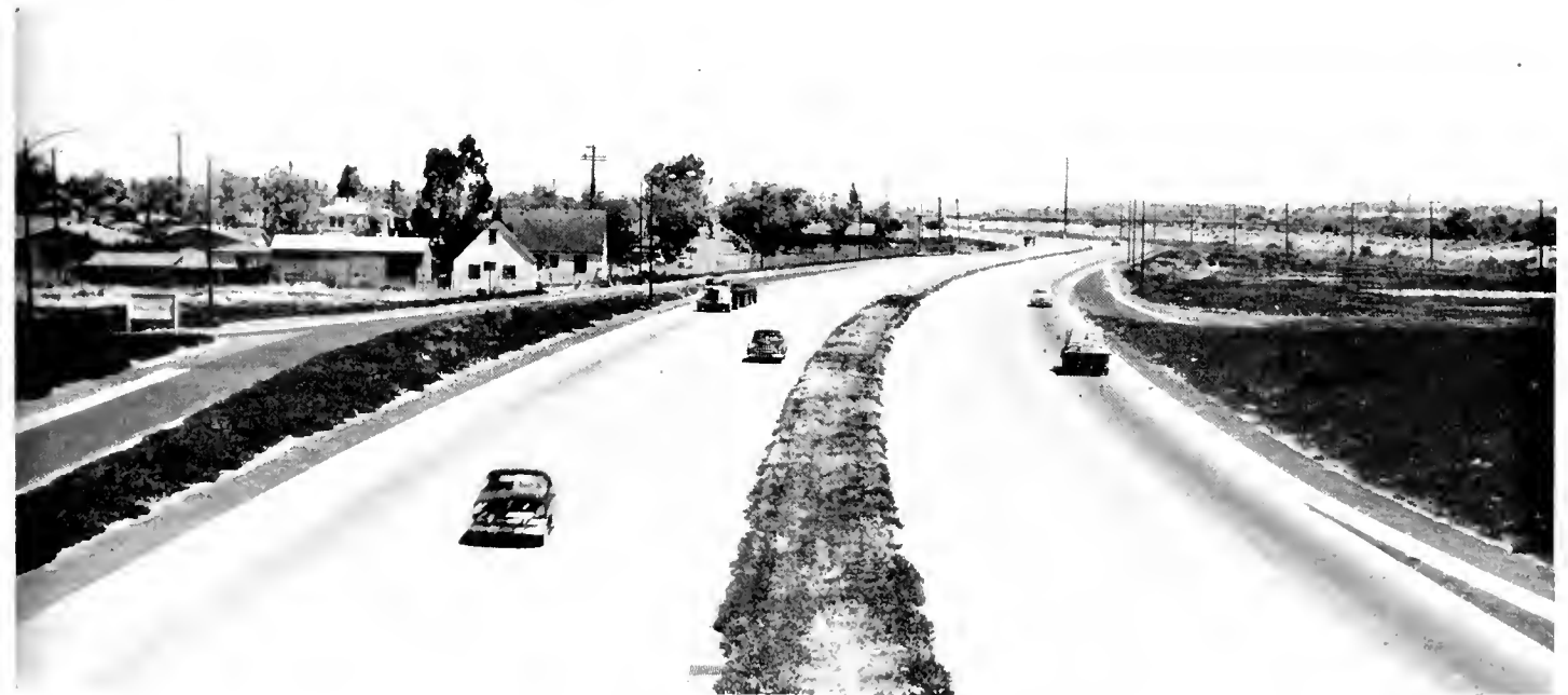
Looking northerly from Pacific Coast Highway along completed section of Long Beach Freeway. Two and one-half miles of this completed construction extends to 223d Street.
